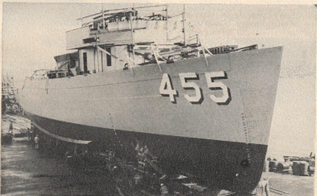
A ship is born. Over 90 percent of the USS Implicit , 171-foot Navy mine sweeper, is constructed of laminates
