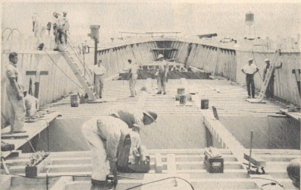
Preassembled transom is fitted to stern. Below, construction scene inside hull as wooden mine sweeper moves to completion
